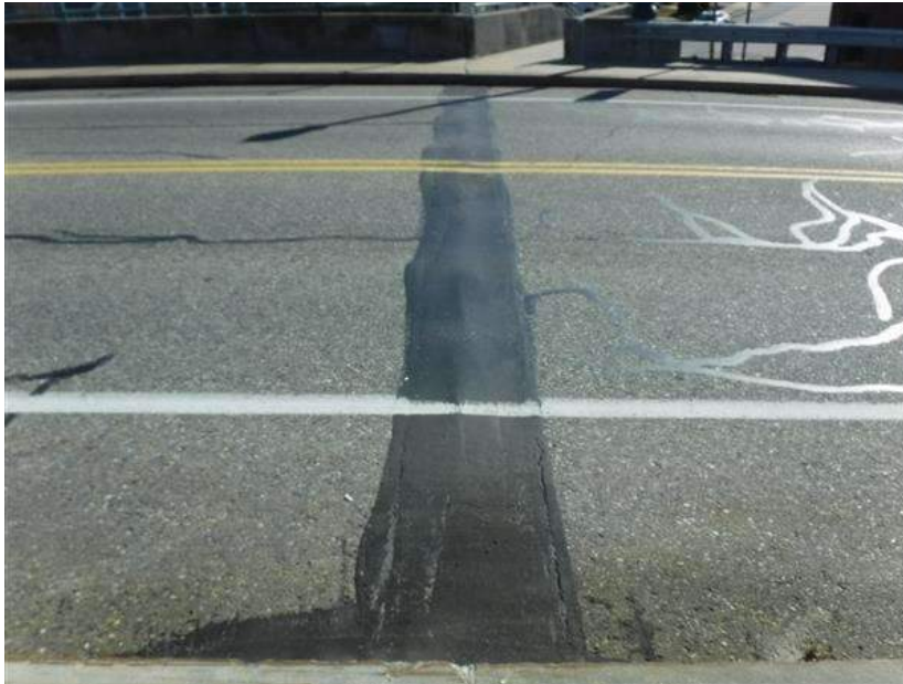
Abutment 1 plug joint has multiple adhesion cracks with full length settlement/depressions, looking east.
