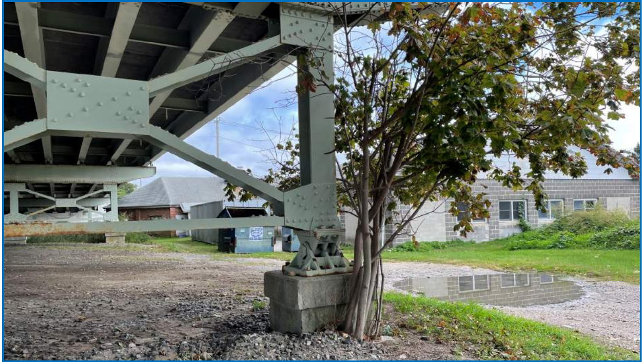
Photo 29: Tree growing beside bearing pedestal under Pier 5.
