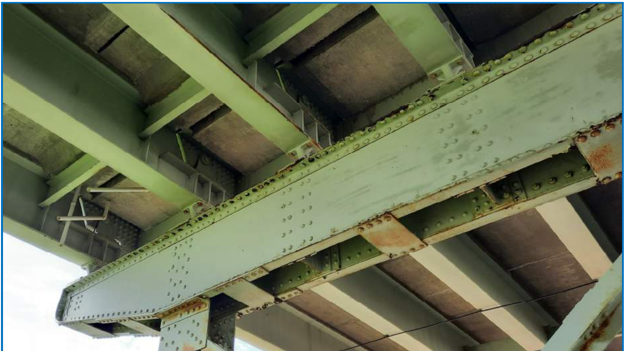
Photo 25: Pier Cap 6 from North side showing top and bottom section losses and random missing rivets..
