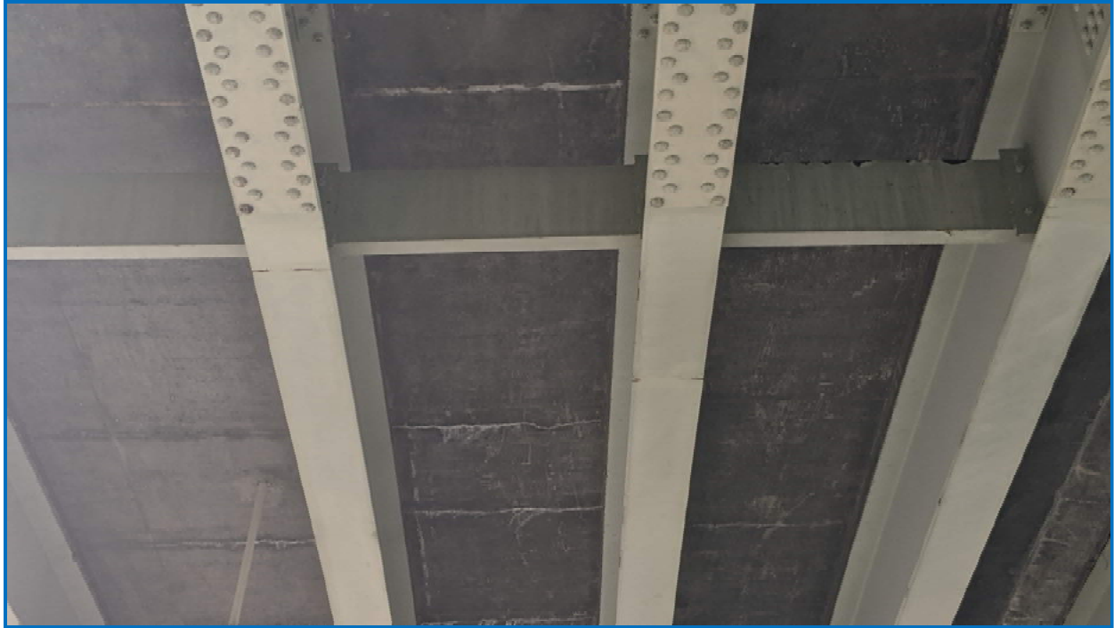
Photo 17: Underside of concrete deck. Random transverse cracks, active efflorescence, and isolated spalling. (Span 6 Girders 8 and 9 in photo).
