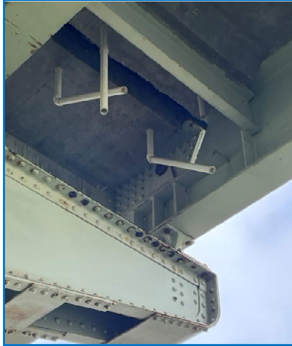
Photo 9: Bridge deck weephole drains extended to prevent drainage onto structure below (location in photo over pier bent 4).
