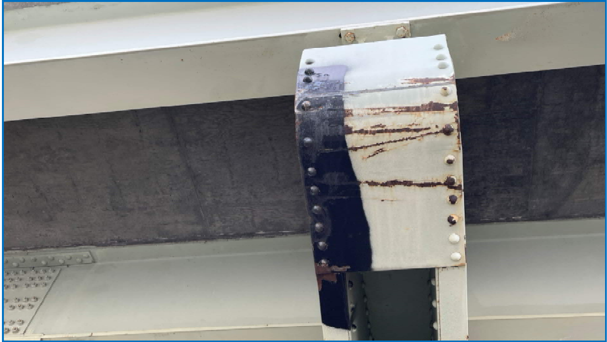
Photo 15: Minor Collision scrape at Pier Cap 3.
