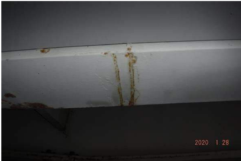
Span 8, Girder G6 bottom of bottom flange near Pier 7 has two (2) impact gouges.
