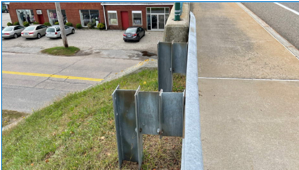
Photo 33: Metal Beam rail with steel posts and block outs. Typical for all approach corners.
