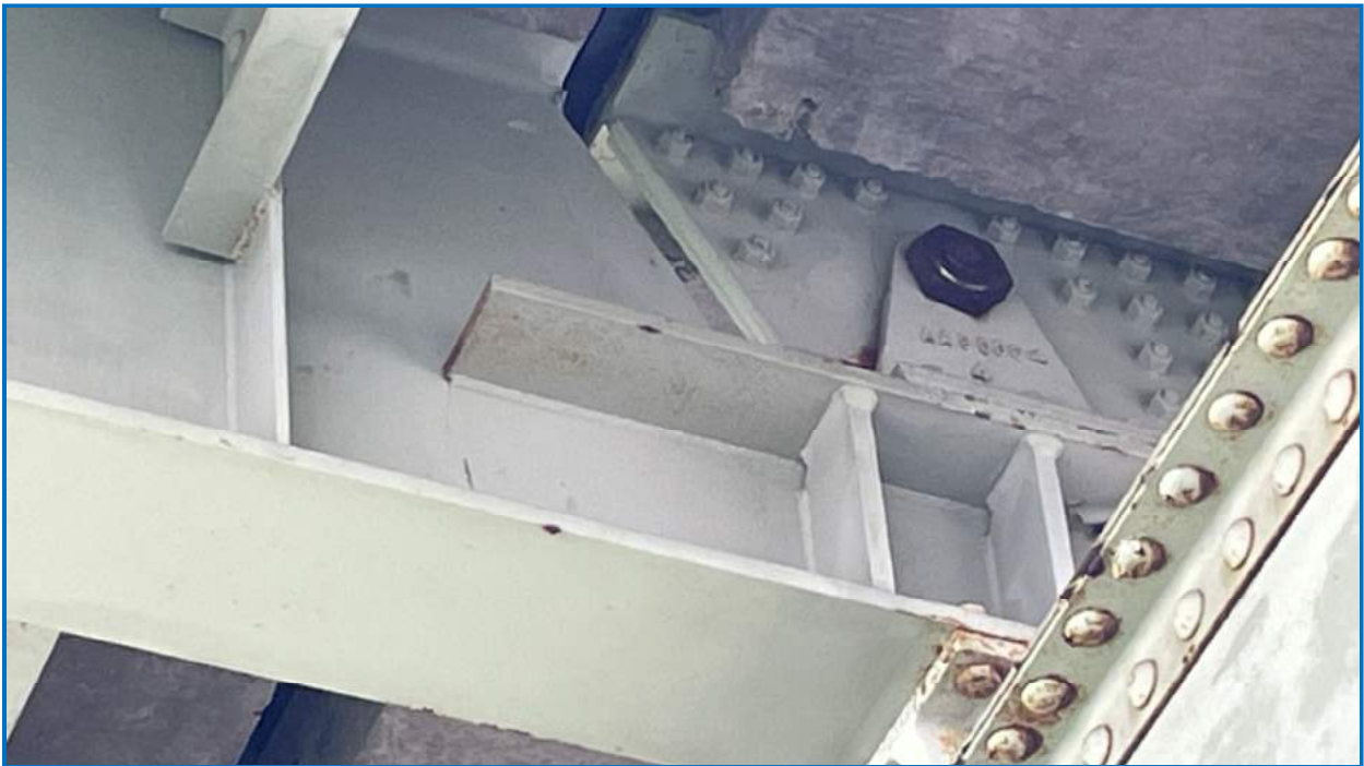
Photo 14: Expansion bearings over pier bent 4. No paint over the nuts or bearing pins (typical).
