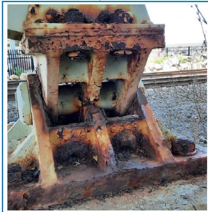
Photo 28: Pier bent bearing under pier 4 showing heavy laminar rust and pack rusting between plates.
