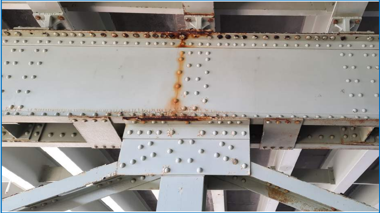
Photo 25: Pier Cap 6 from North side showing top and bottom section losses and random missing rivets..
