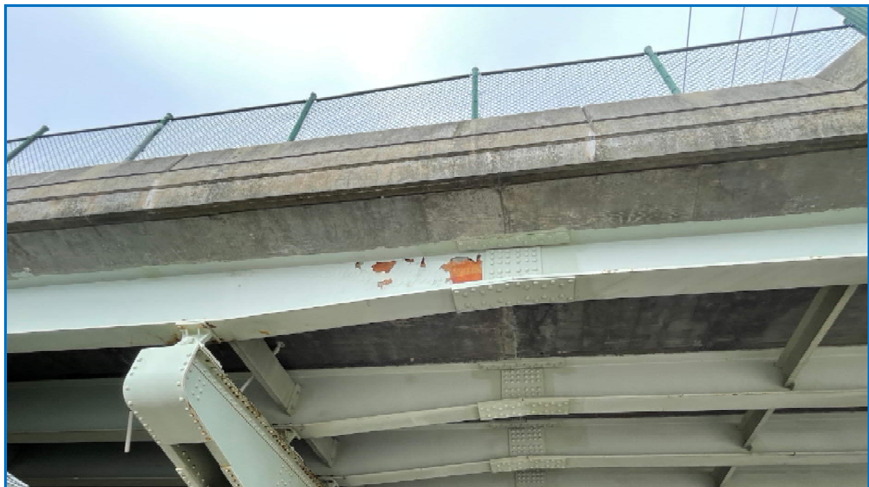
Photo 22: Facia of Girder G9 in Span 8 showing areas of peeling paint and surface rust near field splice.
