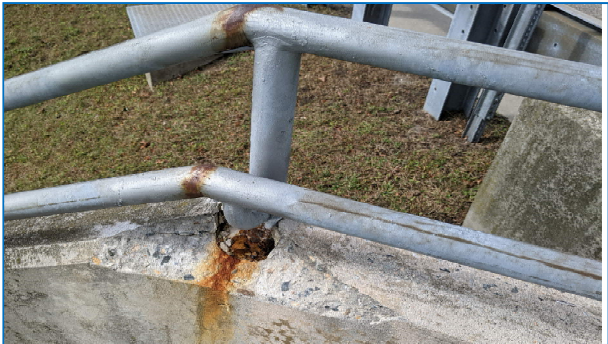
Photo 8: Condition of southeast stairwell showing spalled concrete and missing hand rail post.
