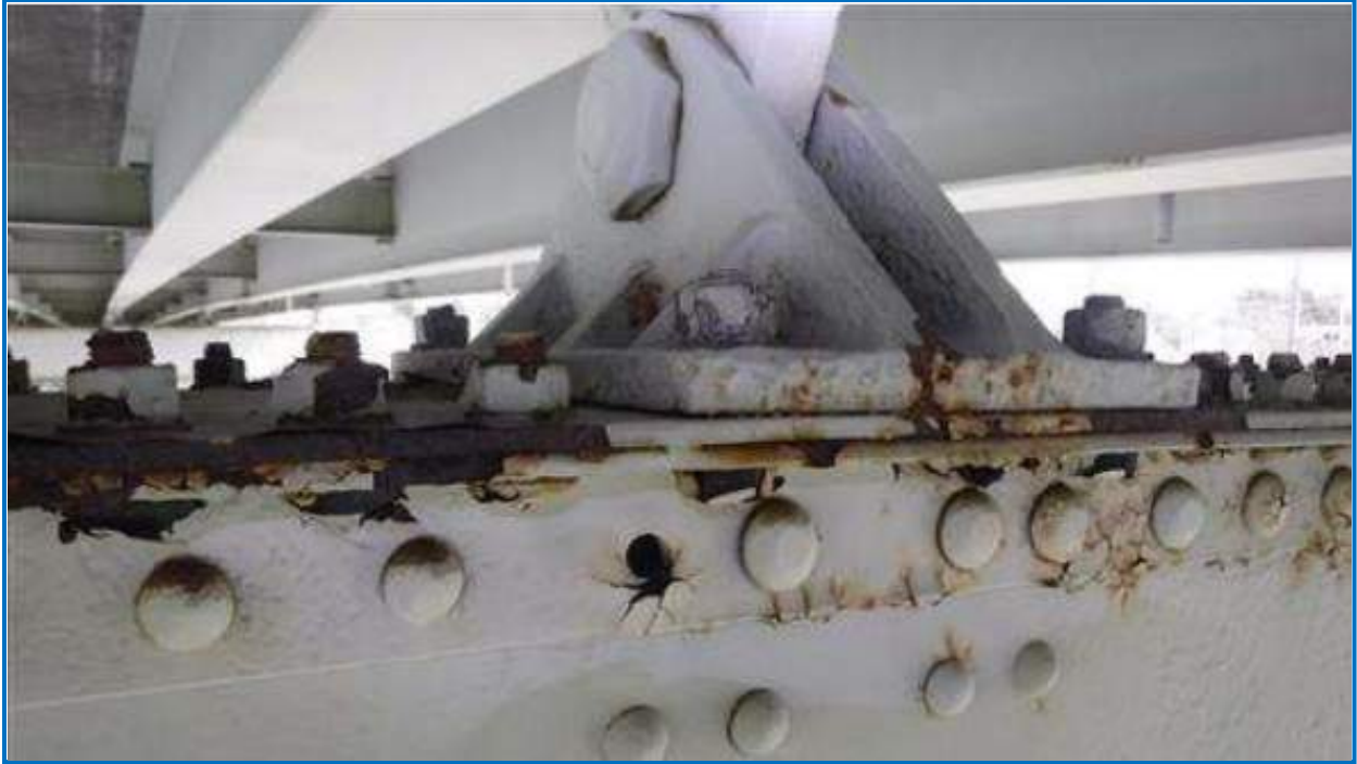
Photo 13: Typical condition of fixed rocker bearings.
