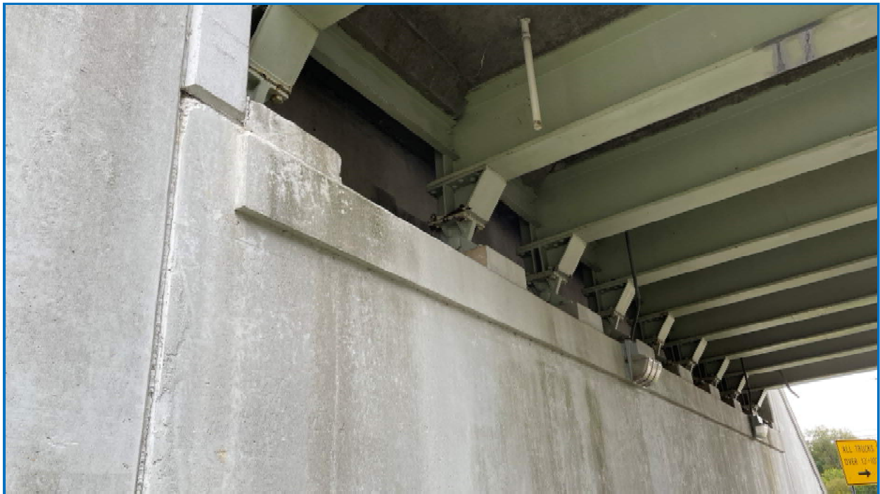
Photo 20: Abutment 2 adjacent to Cutler Street. Note scrape marks on bottom flange of Girder G2 painted over in top right of photo.
