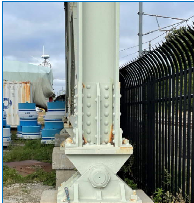
Photo 30: Elevation of Pier 3 column and bearing. Note laminated rust and section losses on interior column legs near bases.
