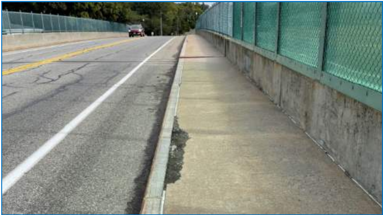
Photo 12: Sidewalk located on south side of bridge (looking North). Isolated areas on sealant and concrete missing behind the granite curbing (typical).
