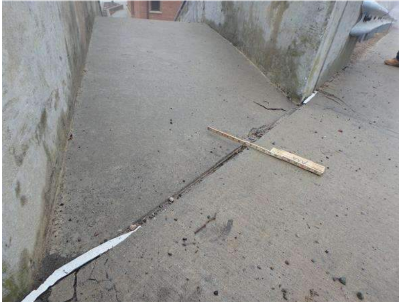
Deteriorated sealant and vertical misalignment at the southeast staircase and southeast approach sidewalk.
