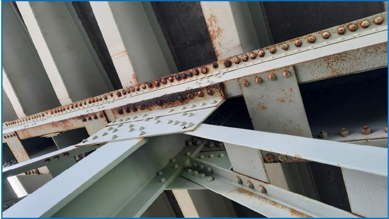
Photo 27: Pier Cap 6 top and bottom flange deterioration over center column. Photo taken from South side of pier.
