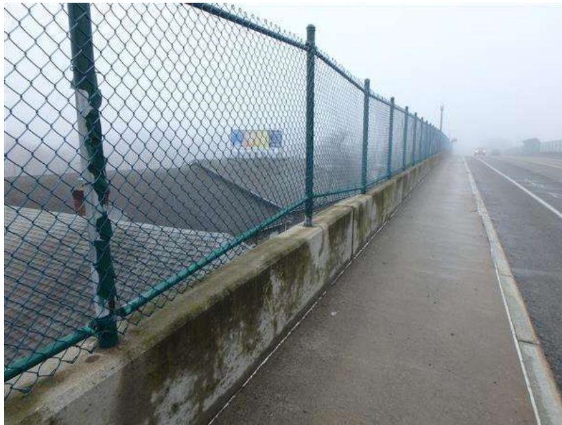
General view of the east sidewalk, parapet and fence. Note the fence post partially lifted out of parapet causing a gap between the fence and top of the parapet in span 7. Also see photo 13.
