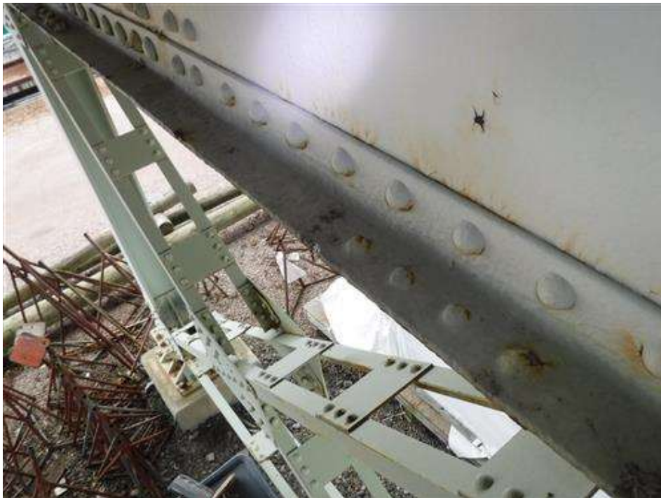
Pier 2 cap, south elevation below Bay 4, the top of the bottom flange angle has painted over section loss and the rivets have up to 50% section loss.
