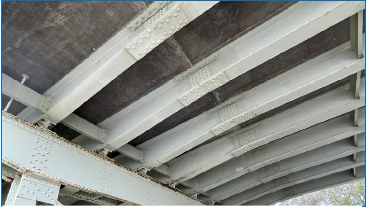
Photo 21: View under Span 8 showing flange transition and field splices adjacent to Pier 7.
