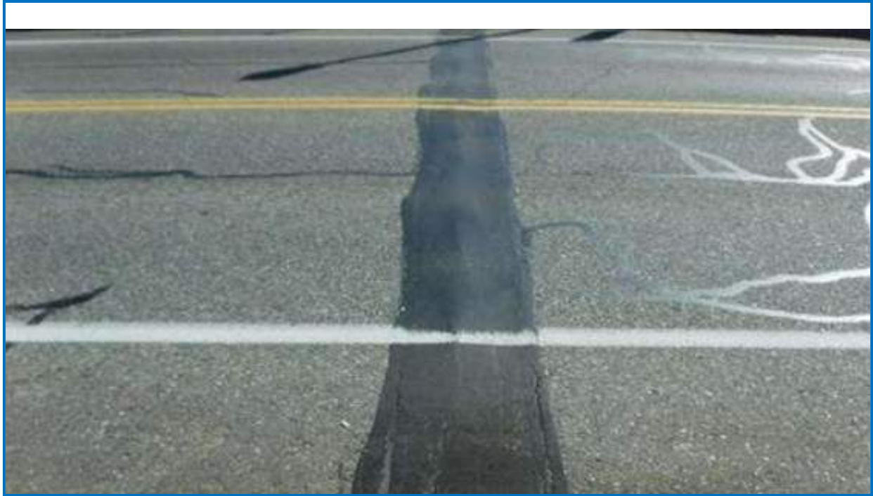
Photo 7: Condition of asphaltic plug joints over abutments. Note adhesion crack and settlement of joints (typical).
