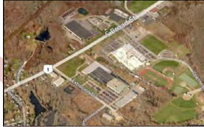
Route 1 @ Extrusion Drive
