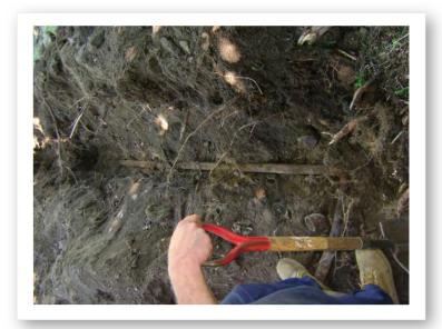
Fuel Line associated with Underground Storage Tank
