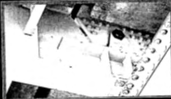
Close up of expansion bearings covered Pier over 4.
