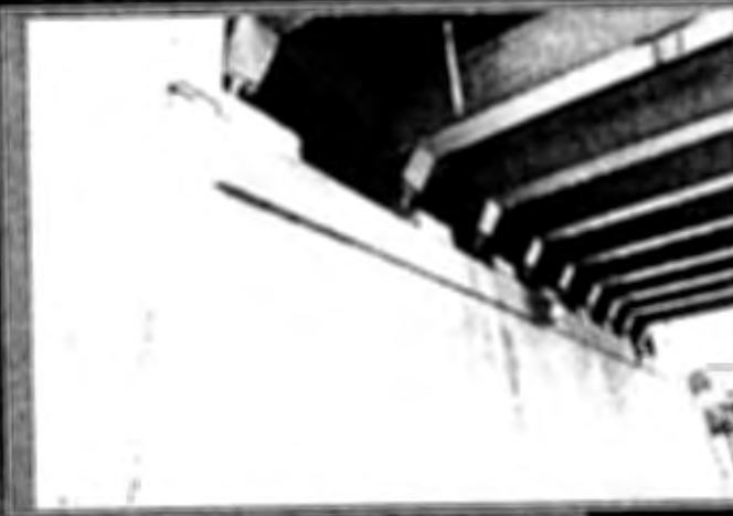
Abutment steelwork (Cyclic Steel) (10015) (10016) (10017) (10018)
