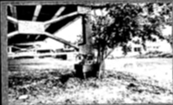
Tree growing beside bearing pedestal under Pier 10015
