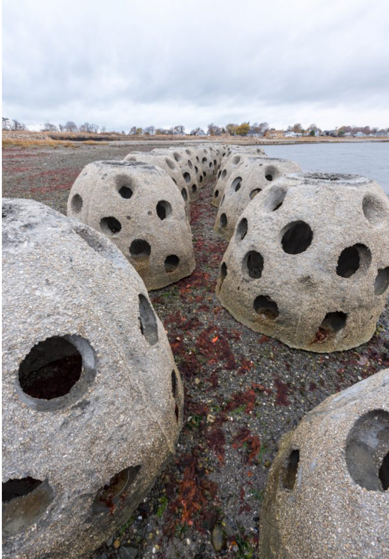
Reef balls line the shoreline of Stratford, Connecticut, protecting the inland with a 35% reduction in wave energy.
