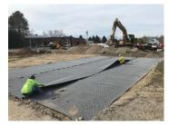
Here you can see the "geotextile" base being installed to support the new **Salt Shed** walls and paving structure. This operation represents an activity necessary to stabilize the ground to support the anticipated 1,100 Tons of salt and heavy machinery to dispense product into Town vehicles. You can see ongoing progress when you drive
