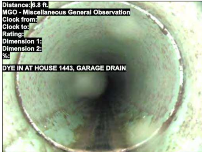
Photo: 1-215-1-212-20221025-091723-092446.JPG At: 6.805 ft. MGO - Miscellaneous General Observation Joint: No DYE IN AT HOUSE 1443, GARAGE DRAIN
