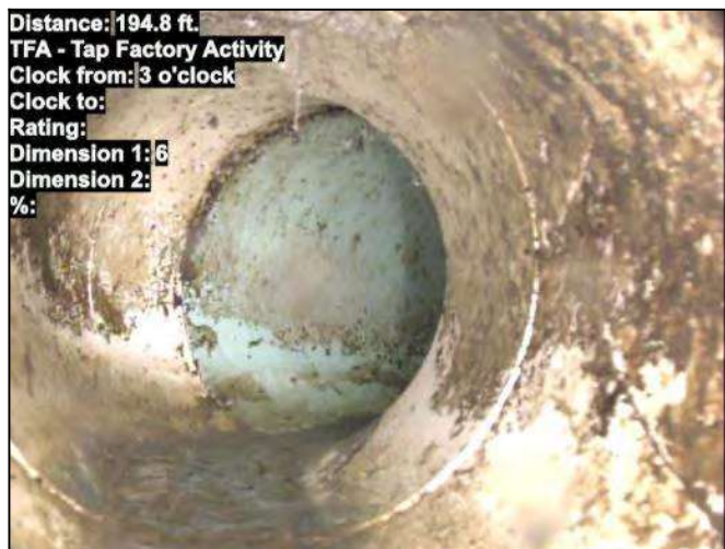
Distance: 194.8 ft. TFA - Tap Factory Activity Clock from: 3 o'clock Clock to: Rating: Dimension 1: 6 Dimension 2: %: Photo: 1-215-1-212-20221025-091723-093453.JPG At: 194.849 ft. TFA - Tap Factory Activity 3/. Joint: No
