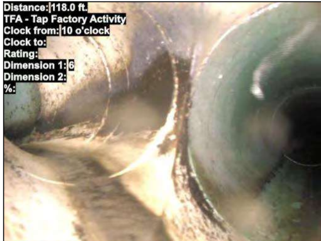
Photo: 1-215-1-212-20221025-091723-093051.JPG At: 117.99 ft. TFA - Tap Factory Activity 10/. Joint: No
