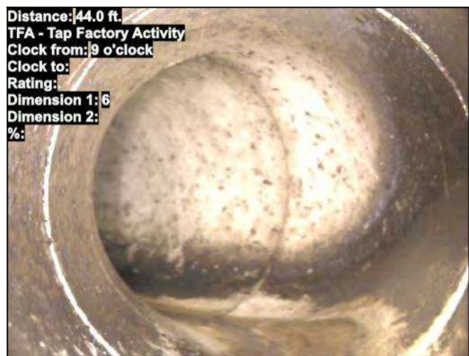
Photo: 1-229-1-228-20221025-102314-103635.JPG At: 44.034 ft. 9/. TFA - Tap Factory Activity Joint: No
